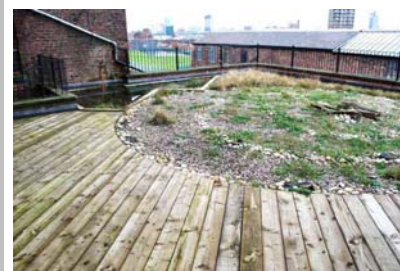
Photo 9: Purpose built roof, MERCI, Ancoats, Manchester
