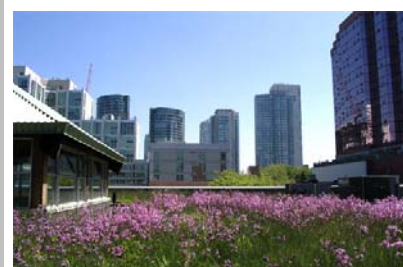
Photo 23: Mountain Equipment Co-op green roof, Toronto
