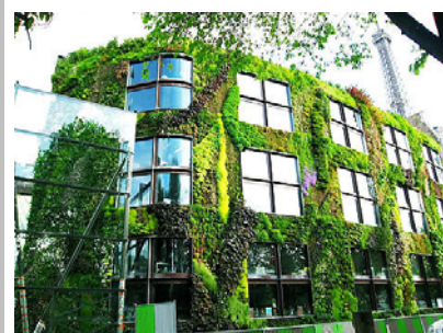
Photo 12: A 'living wall' in Paris – a Patrick Blanc wall, Musee du Quai Branley .
