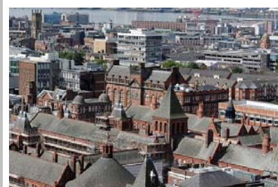
Photo 4: A ‘grey’ roofscape across Liverpool rooftops towards the River Mersey.
