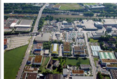
Photo 25: Aerial view of green roofing, City of Linz
