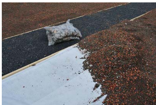
Pond with waterproof liner and other biodiversity features being installed:
