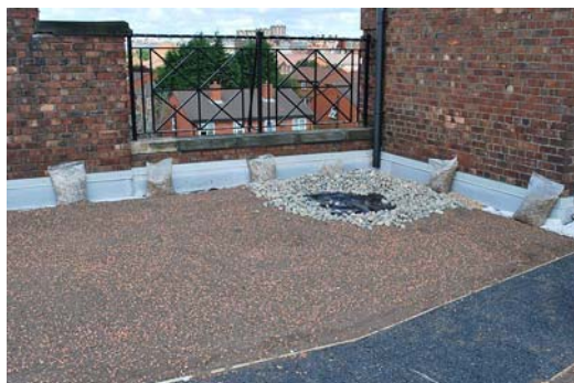
Pond with waterproof liner and other biodiversity features being installed:
