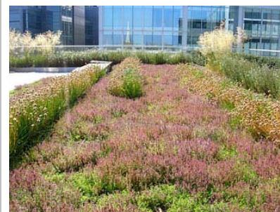
Photo 19: Intensive green roof, London
