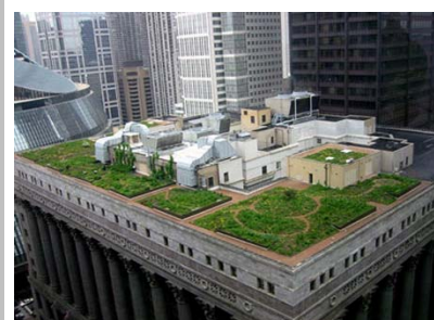
Photo 10: Chicago City Hall.
