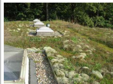
Photo 3: A green roof, Okowerk Environment Centre, Berlin - 1890
