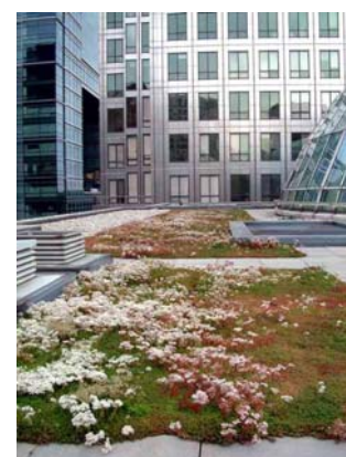
Photo 5: A view onto a Sedum roof in Canary Wharf, London
